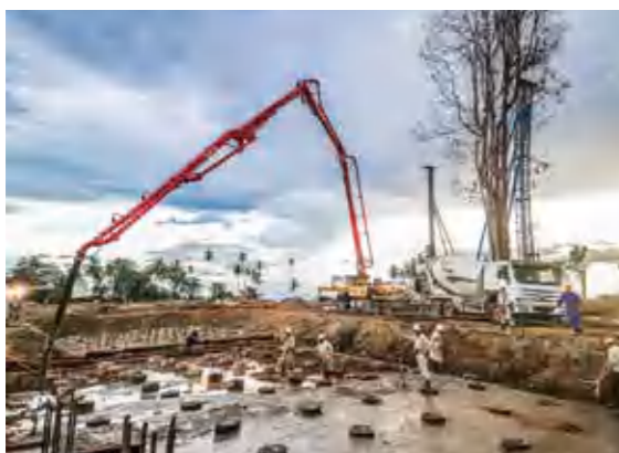
徐工泵车助力印度尼西亚 XCMG boom pump is working in Indonesia.
