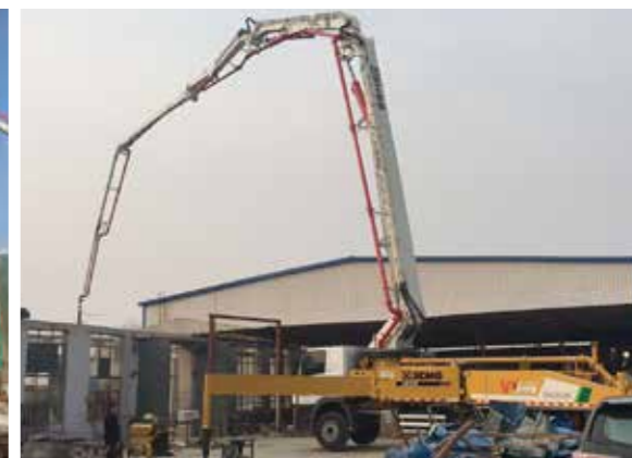
徐工泵车哈尔滨小试牛刀 XCMG boom pump is trying its hand in Haerbin
